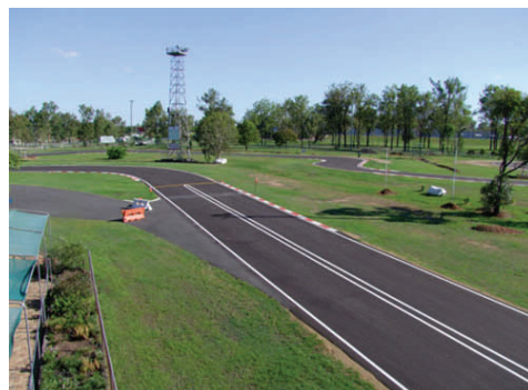
Ipswich's re-surfaced track is ready for action
